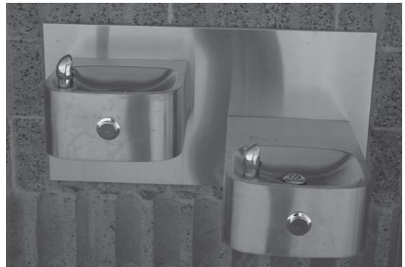
Fountains Connected to a Central Chiller
