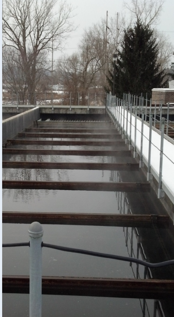
Effluent energy recovery
