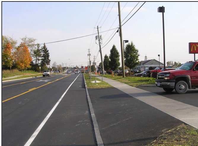
Recently Improved Driveway and Sidewalk Along Arterial Street
