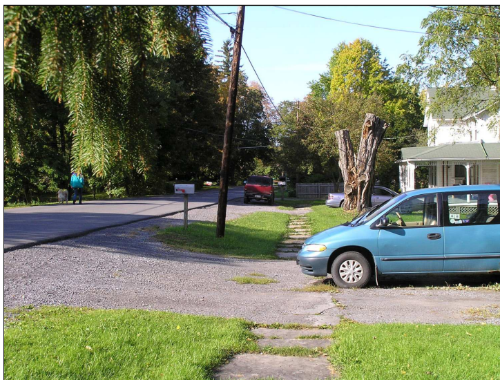
Tree Lawn Area that Needs Improvement
