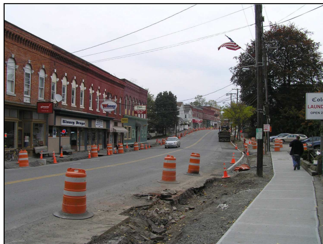
Main Street Under Construction
