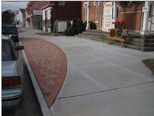
Main Street Sidewalk Improvement
