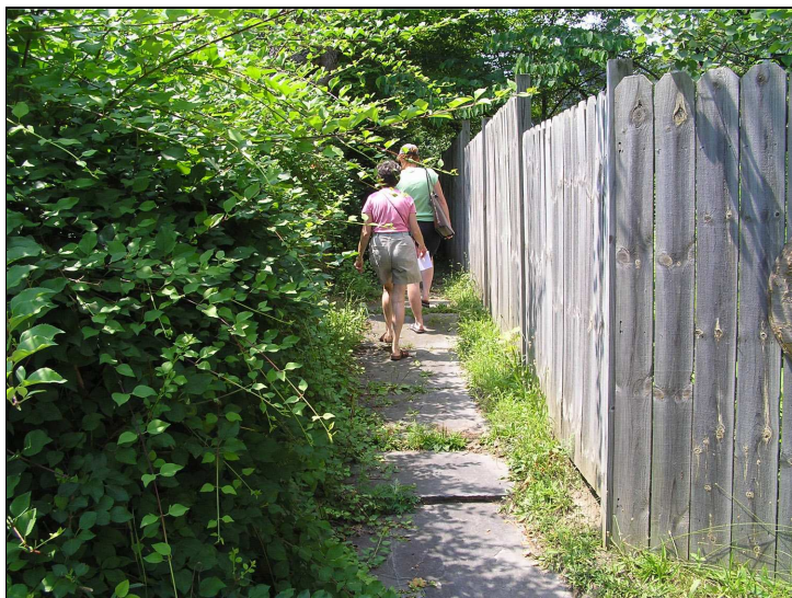
Brush Overgrowth between Street and Sidewalk
