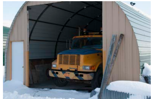
Quonset Hut Truck Storage at Ithaca NYSDOT Maintenance Facility (Fisher Associates)
