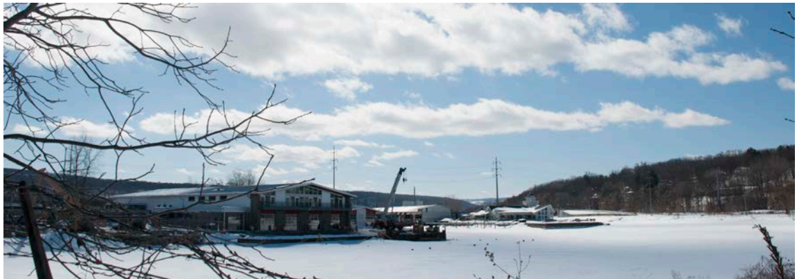
Cornell University Boat House (Fisher Associates)
