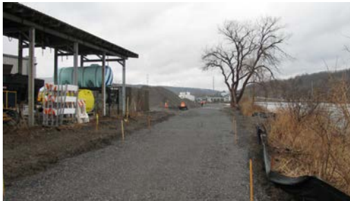
Cayuga Inlet Trail Extension Under Construction (Fisher Associates)
