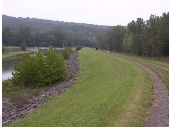
Figure 5.4.4-1. Cayuga Inlet Levee System
