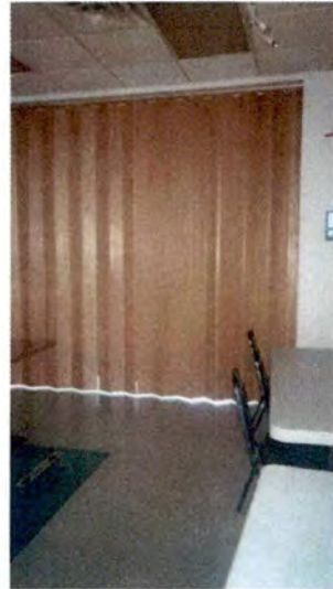
View of Barrier outside of smoke room showing gap at bottom
