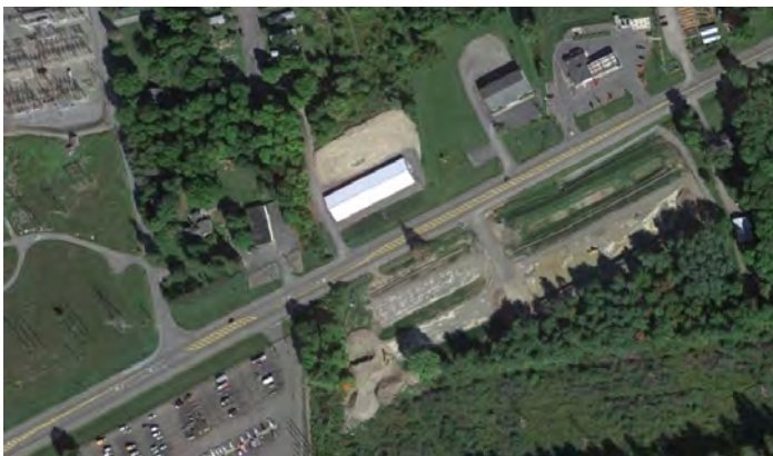
Driveways near the NYSEG property
