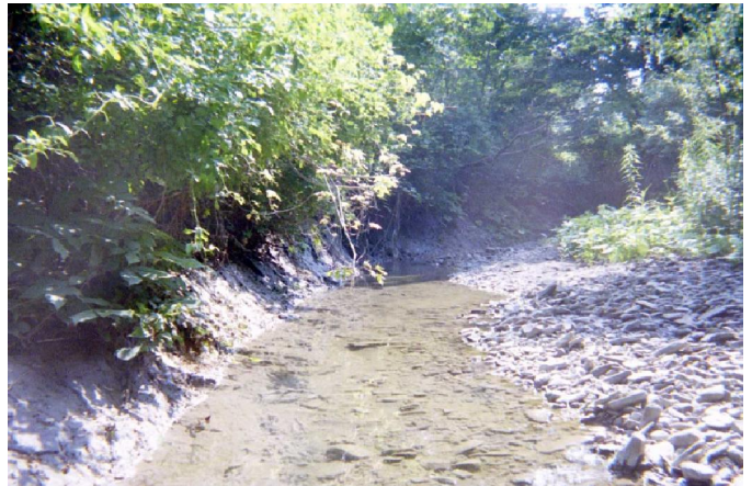
Erosion along Sixmile Creek is a major concern. Several studies reveal that this erosion is largely the
