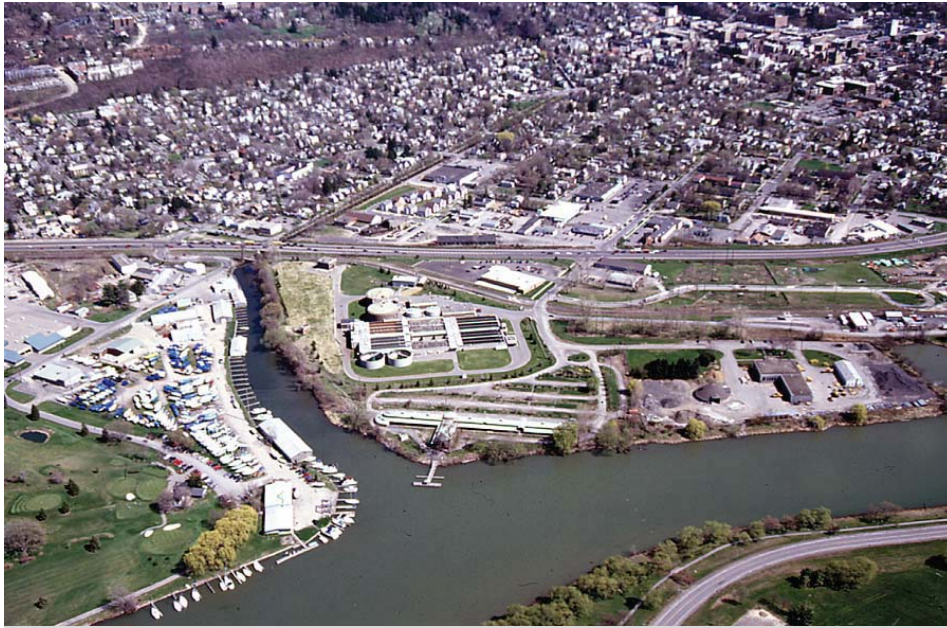
Cascadilla Creek as it enters the Inlet. Johnson's Boatyard, Steamboat Landing (Farmers' Market) and a DOT maintenance facility occupy the Inlet's east shore.
