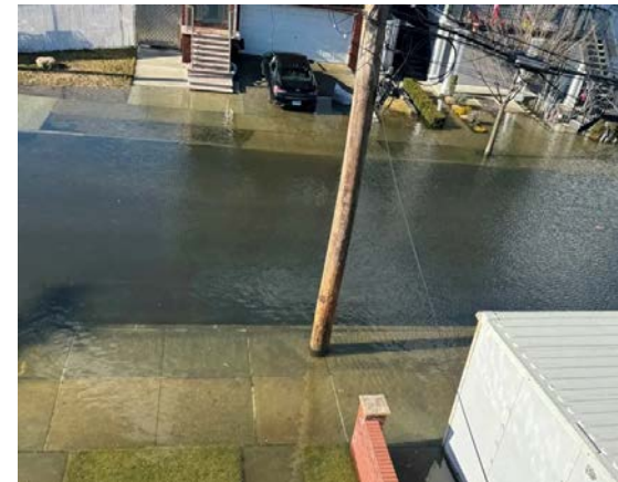
Impassable roads due to floodwater
