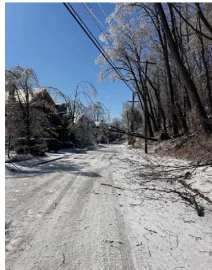
Downed trees & powerlines (be careful)
