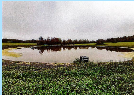
Constructing Retention Ponds
