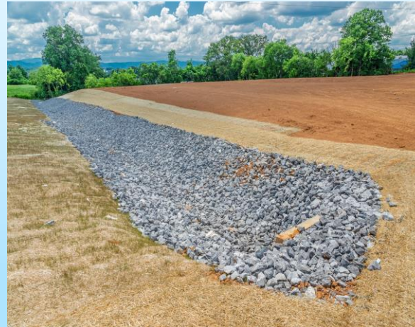
Lining Ditches and Streams
