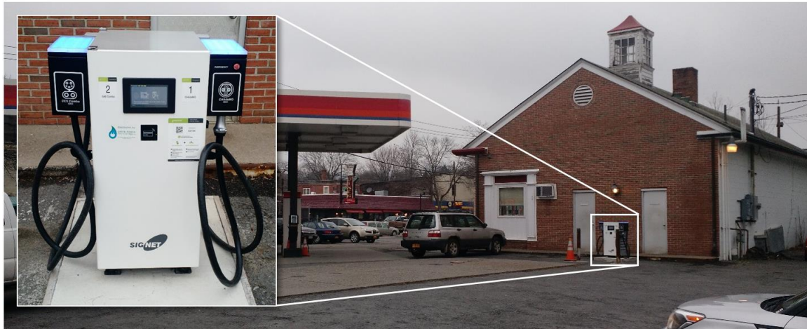
Figure 11: DC Fast Charger Installed at Diane's Downtown Automotive
