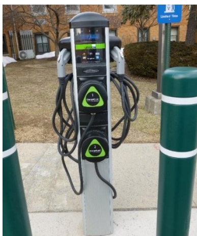
Figure 7: AC Level 2 Charging
