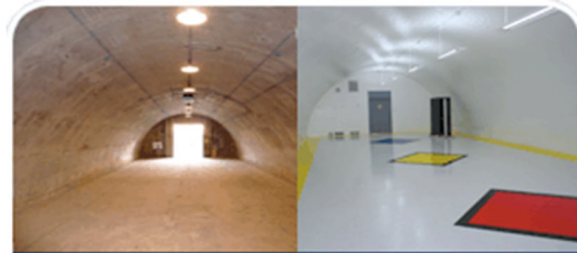
BUNKER INTERIOR - BEFORE AND AFTER
