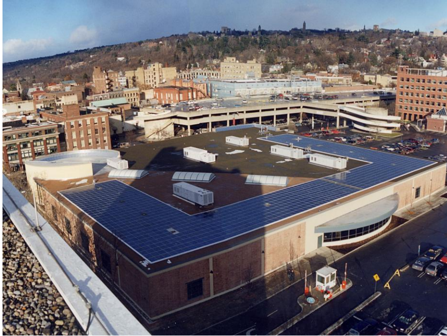
Figure 26: Photo of the Tompkins County Public Library taken from the roof of the Holiday Inn across the street. Notice the shadow of the hotel blocking a significant portion of the solar panels from sunlight. This is a problem that should have been foreseen and avoided.
