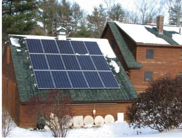
Figure 9: Roof mounted PV system. Notice the lack of trees and other obstructions that could potentially shade the panels. Also notice the slope of the panels allows snow to slide off instead of accumulating.
