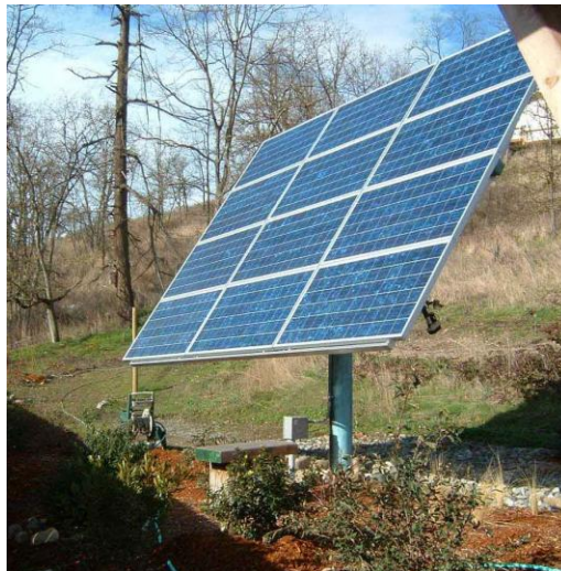
Figure 10: Ground mounted PV system. The tilt of the array can be adjusted from the ground to adapt to different seasonal sun conditions.
